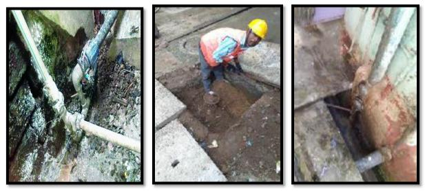
Fig: 8 Water pipelines leakage and connection stealing (Quaterly newsletter from NCDC)
